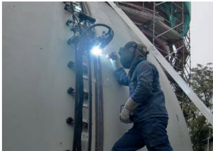
Pipeliner mounted on Flx-Track in 3.3m (11 ft.) diameter duct
