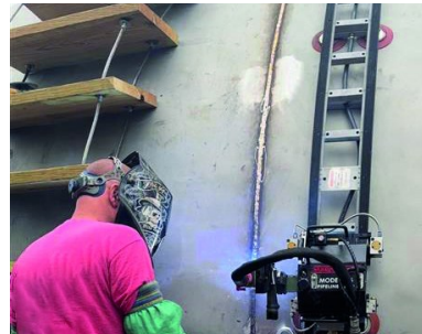
Pipeliner mounted on a stainless steel vessel using vacuum cup kit
